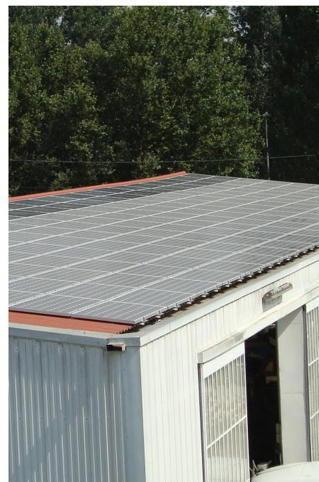
ESV Energie, a French-American company which specializes in implementing energy efficiency projects across Europe, acquired a 34 kW system in the French town of Tarascon. The installation at Tarascon is made up of 6 x SolarEdge SE6000 inverters and 200 Trina Solar 180W monocrystalline modules with SolarEdge power optimizers. It is meant to serve as a long term financial investment.
