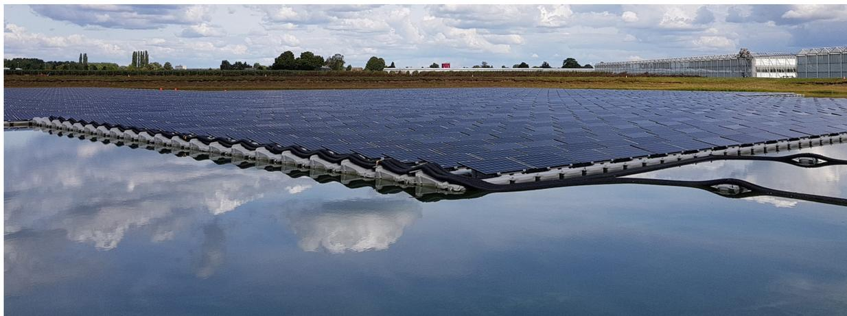
Located in a Netherlands irrigation water basin, the 1.845MW Lingewaard Floating Solar Park took an expanse of water and, in conjunction with SolarEdge, turned it into a green energy power source. Installed by Tenten Solar, the field produced 1 million kWh of energy from 6,150 panels, barely five months after installation on 31 August 2018.
